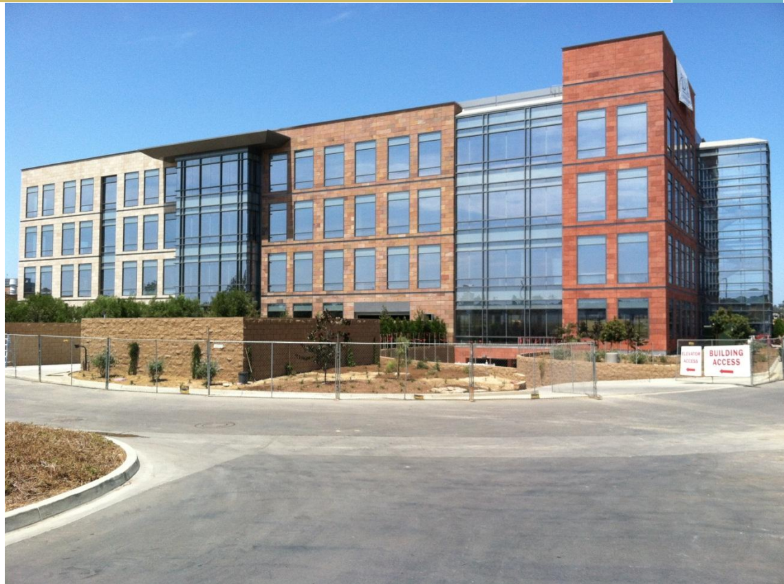
Figure 1: View of Building, Maffett
